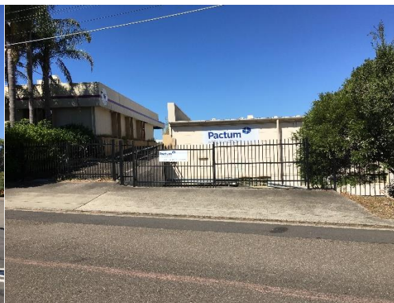
Photo 6: View of existing loading dock accessed from Kareena Road to building at 142 Parraweena Road
