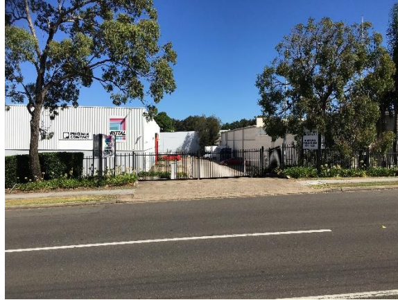
Photo 2: View of existing building and loading dock at 130 Parraweena Road.
