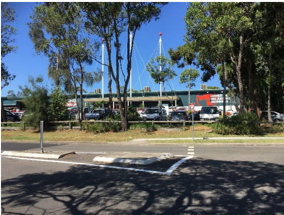
Photo 17: View of existing Bunnings development at 31-35 Willarong Road.
